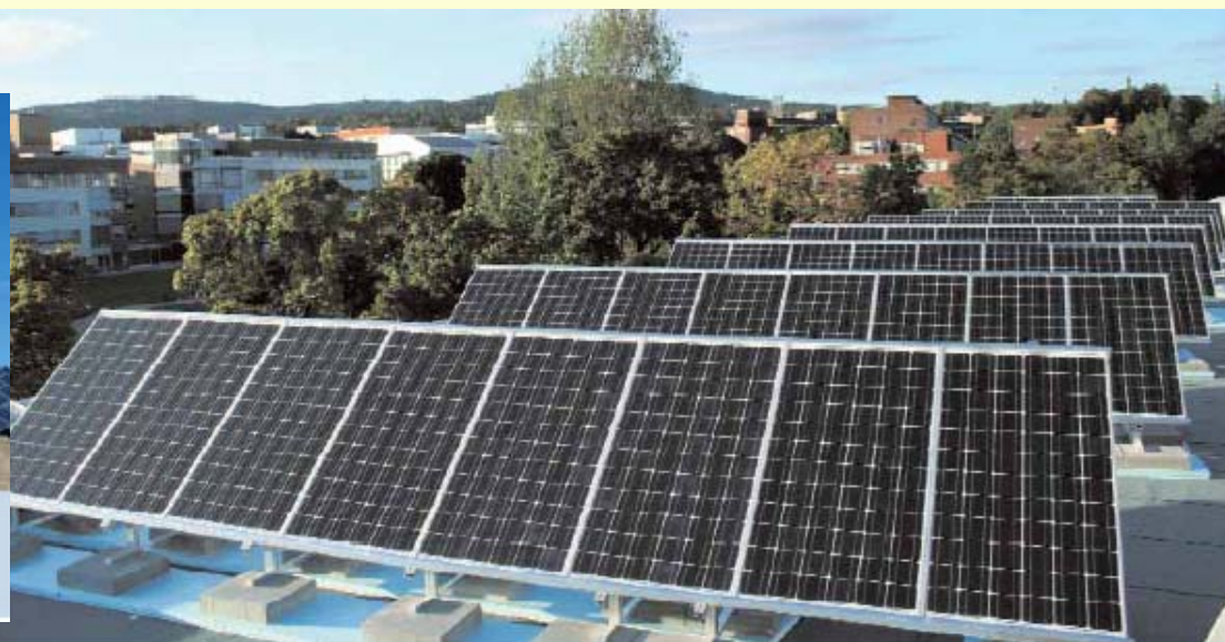
Fig. 1 - The 17,6 kWp installation on the roof of Oslo Innovation Centre in Oslo (photo Norsk Solkraft as).
